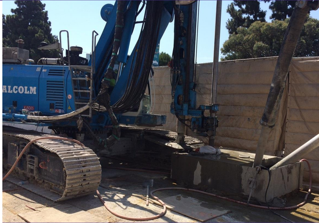
Example of jet grouting at Wilshire Bl/Highland Av
