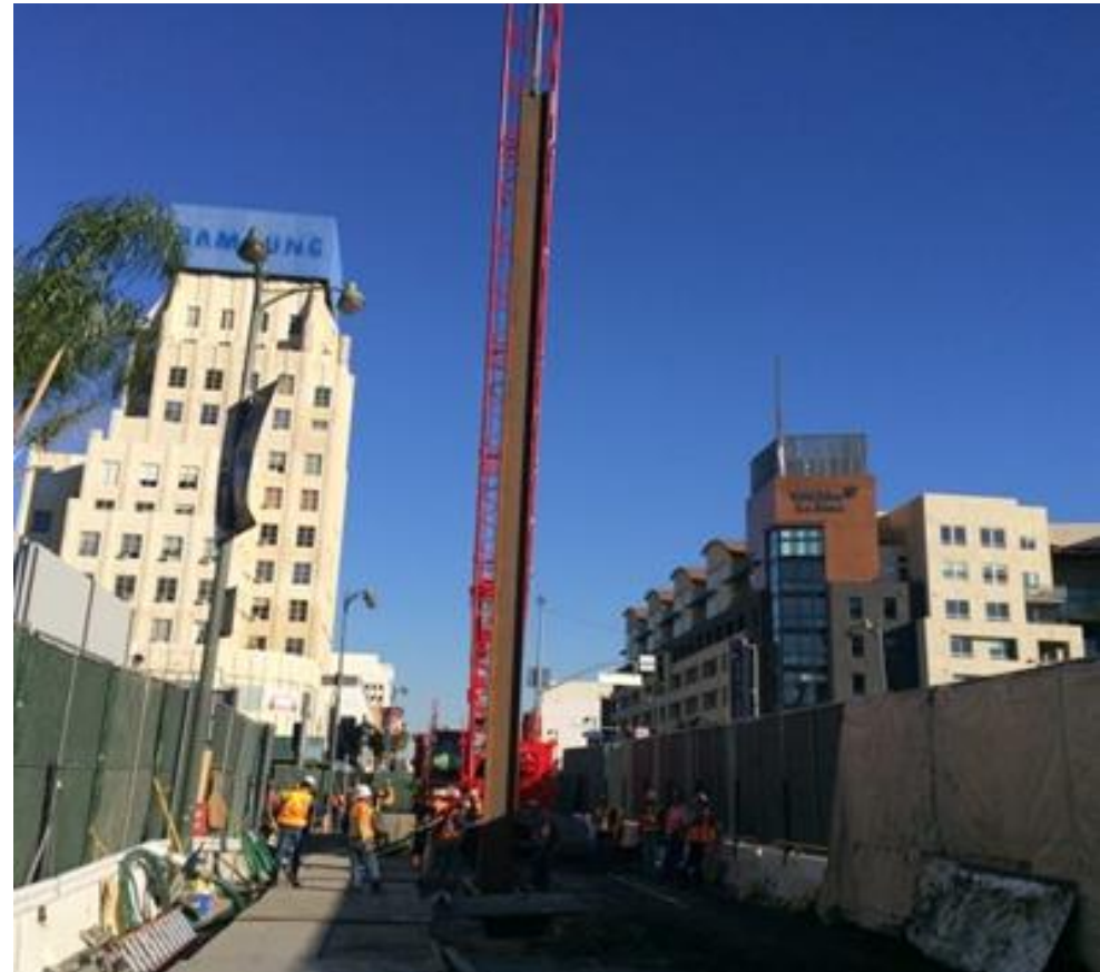
Typical pile installation west of La Brea Av on Wilshire Bl
